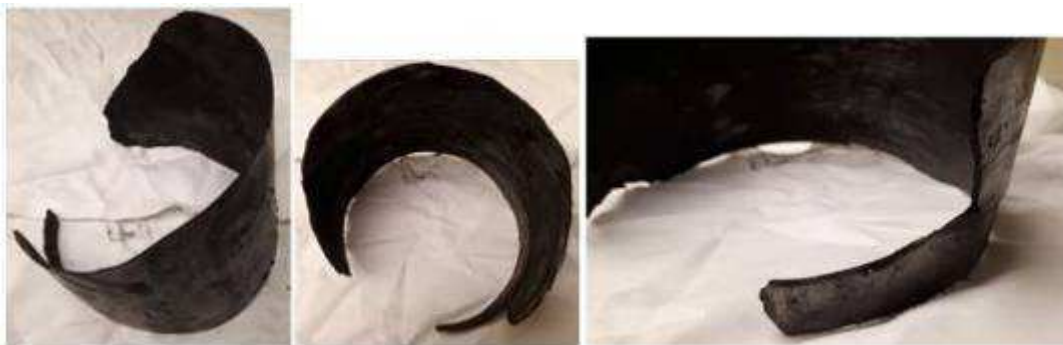
Image 4: Metals spray coating that was under the 1 st Intermediate shaft gear. This failed initially at the metal spray coating at the keyway.
